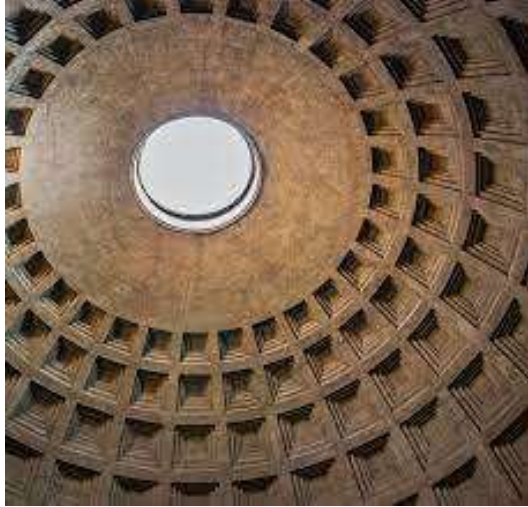
Figure 5: Above ( https://en.wikipedia.org/wiki/Coffer ) we see an example of a coffer in building architecture, which is a series of (square) sunken panels.
